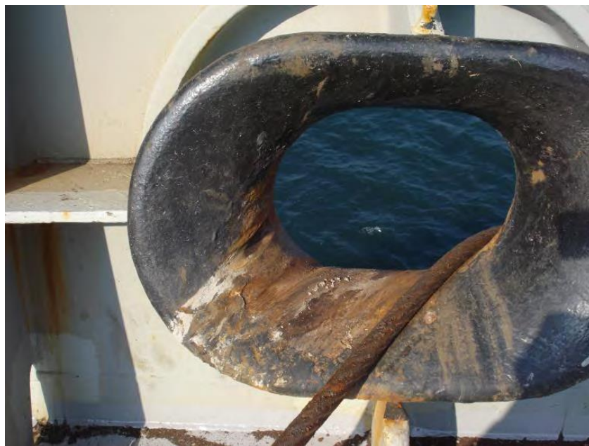
Figure 2 : Closed chock and wire not properly greased
